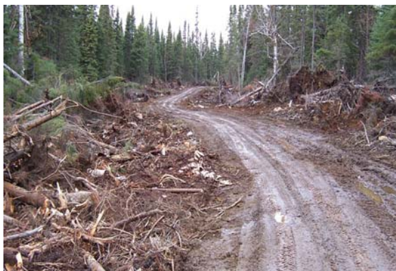
Example of a road built on Crown land
